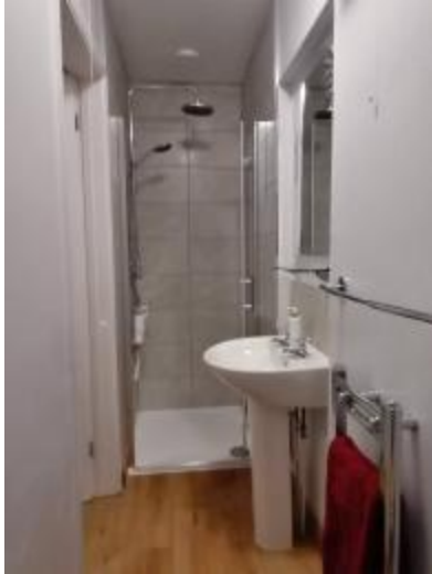
Shower with bifold internally opening door. Small (2cm) step up. Pedastal basin.
