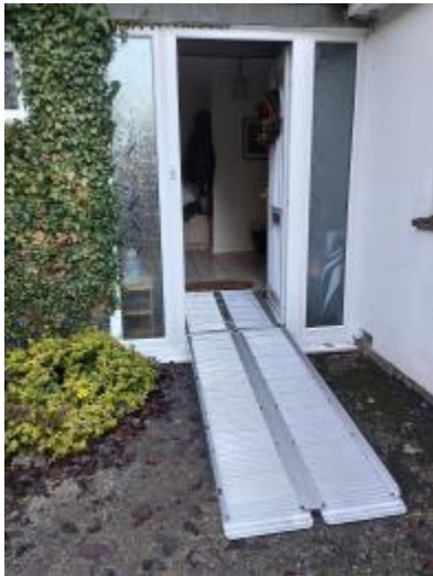
Main entrance with portable wheelchair ramps in place
