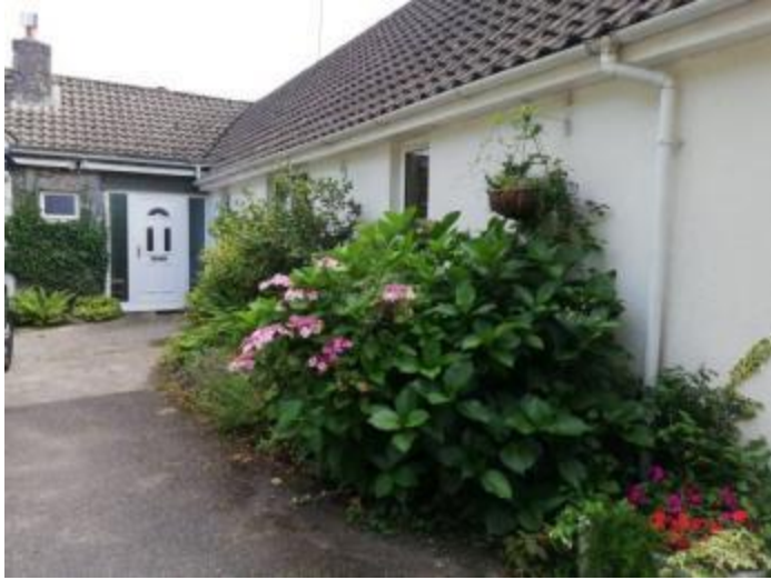
Driveway and main entrance
