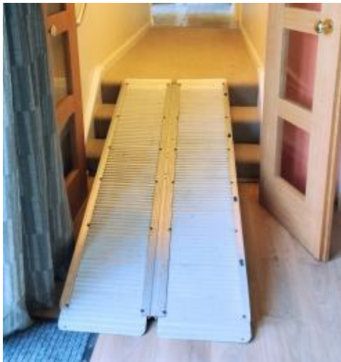
Portable wheelchair ramp from entrance hallway into guest lounge and dining area
