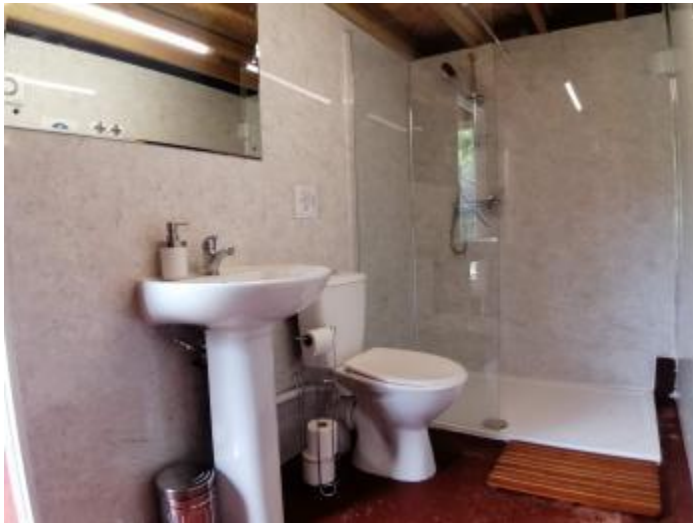
Campsite shower room. Shower with 2 cm high tray. Toilet and pedestal basin
